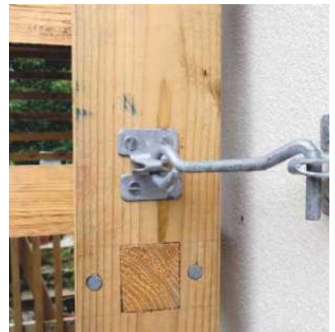
... and the hooks and eye stop the shed moving against the house
